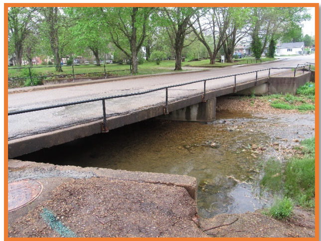
(Mine Street Bridge in Potosi, MO)
