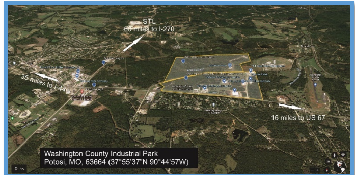
(Aerial of Washington County Industrial Park)
